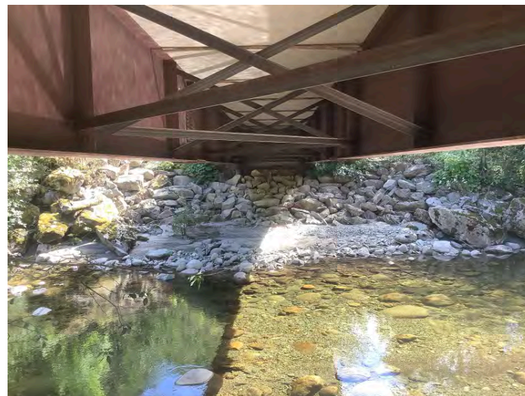
Left Bank Abutment when facing downstream
