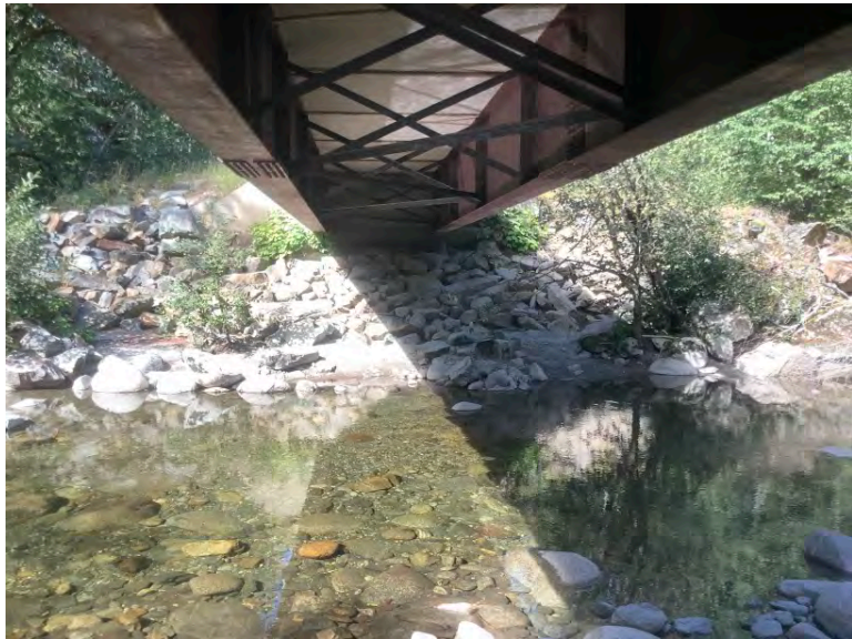
Right Bank Abutment when facing downstream
